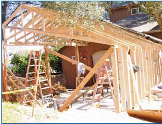
New shower/restrooms framed in
